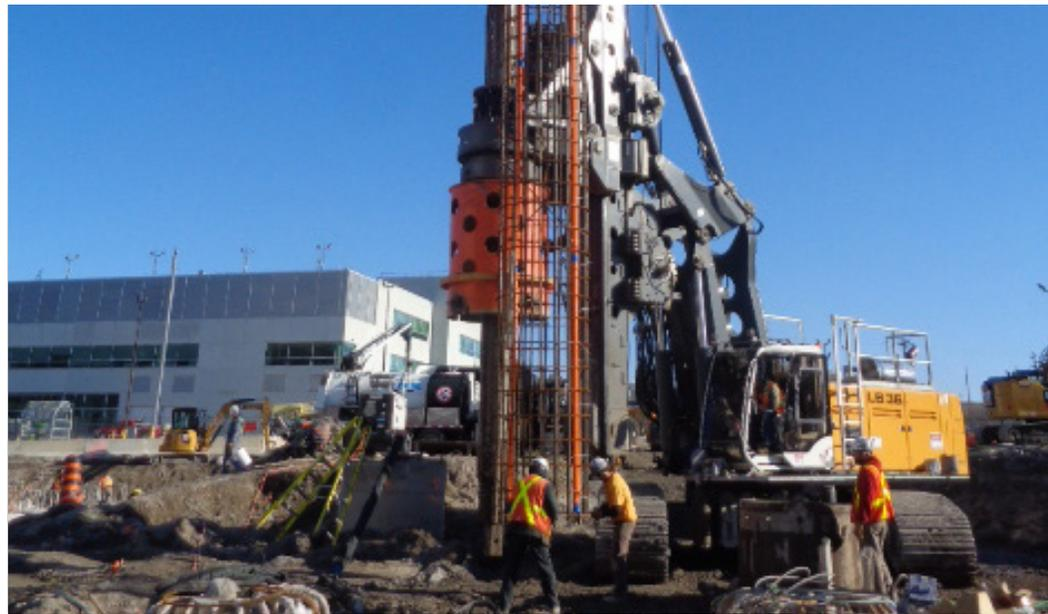
Installing the cage assembly
